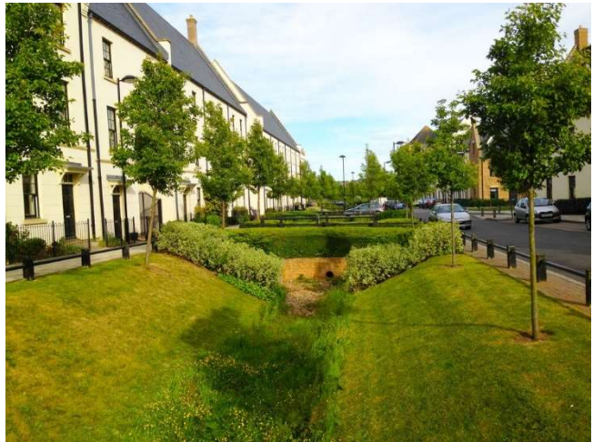
Upton street swale
